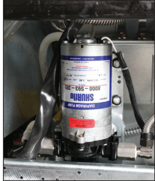
A 24-volt pump moves the oil from the JIB to the frypots. The pump is accessible from the rear of the fryer. It is mounted vertically or horizontally, depending on the space available in the fryer cabinet.
